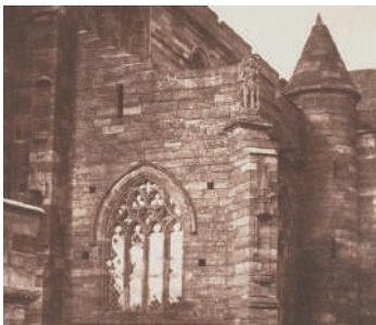
A mid-19th-century photograph showing a mutilated St Michael and empty niches.
