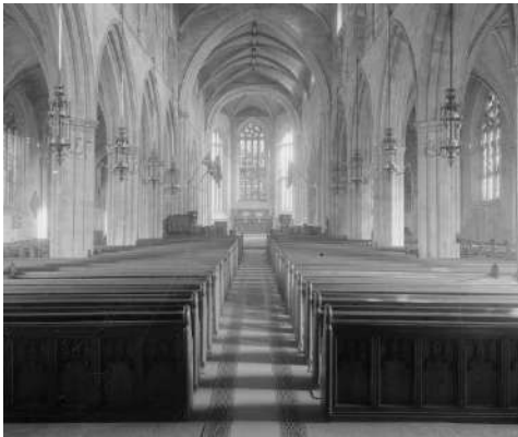
The new seating installed
