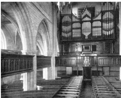
The galleries before demolition; the Royal Pew in the rear centre.
