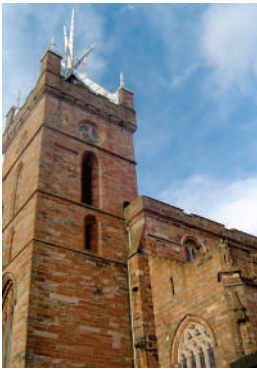
Empty statue niches and the damaged figure of St Michael.
